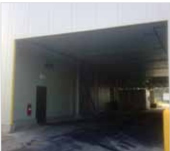
Opening to Fill Tunnel
