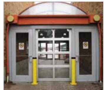
Swing Doors and Aluminum Sectional Door
