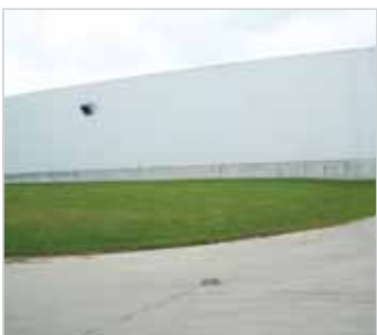
Before Wall Cut-Out
