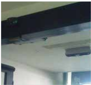
Approach Side Sensors
