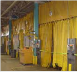
Plastic Sheeting Before
