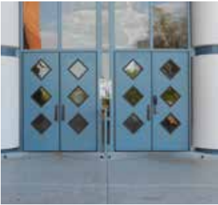
FRP Door After
