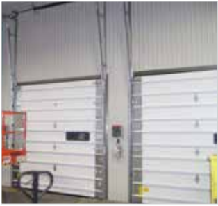
Insulated Sectional Doors After
