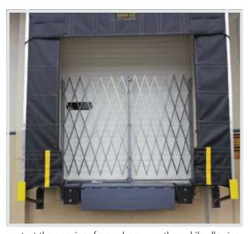
protect the openings from adverse weather, while allowing unobstructed access to the full width of different size trailers. The new dock system has increased the capacity to move materials in an out of the facility, improved employee safety, and with the addition of the scissor gate been able to add more security while the door is open for ventilation.
