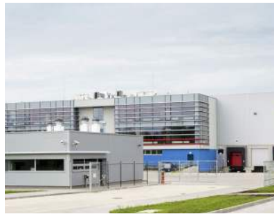
INDUSTRIAL AND MANUFACTURING
